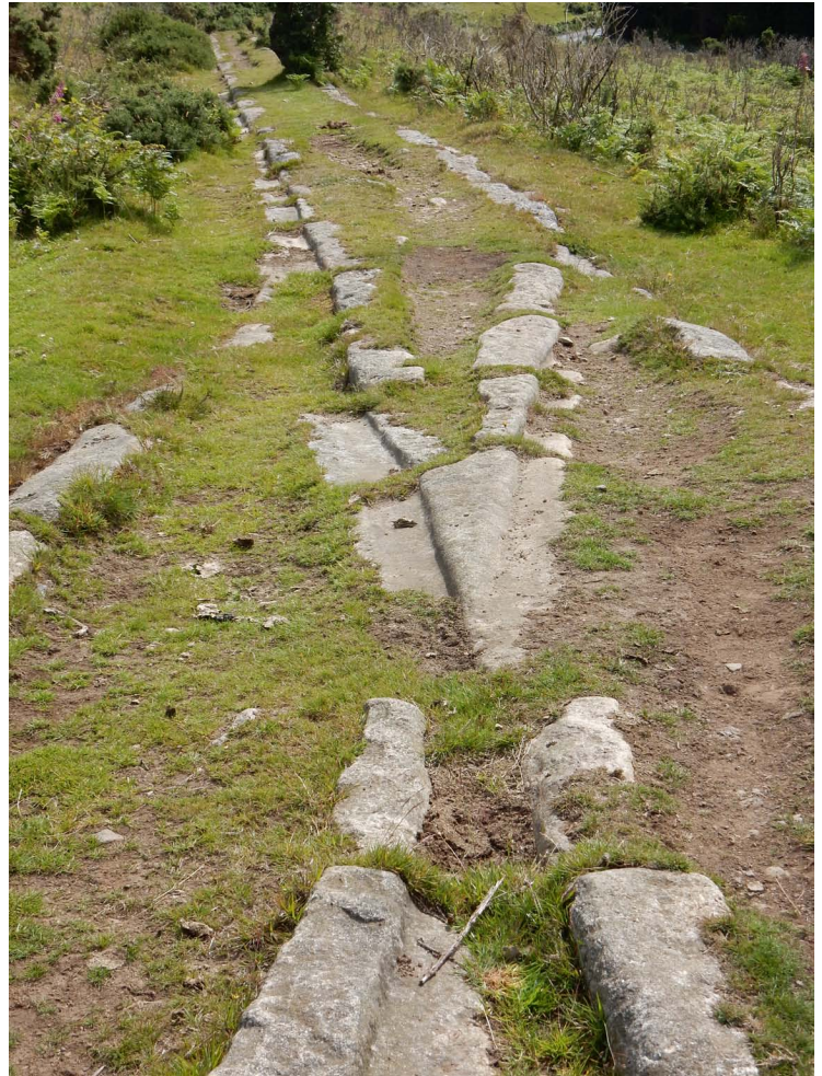
The earliest railways made use of wooden rails, but a few systems used stone before iron became near-universal in the first decades of the 19th century. This is the Haylor system in Devon, built in 1820. © Neil Cossons
