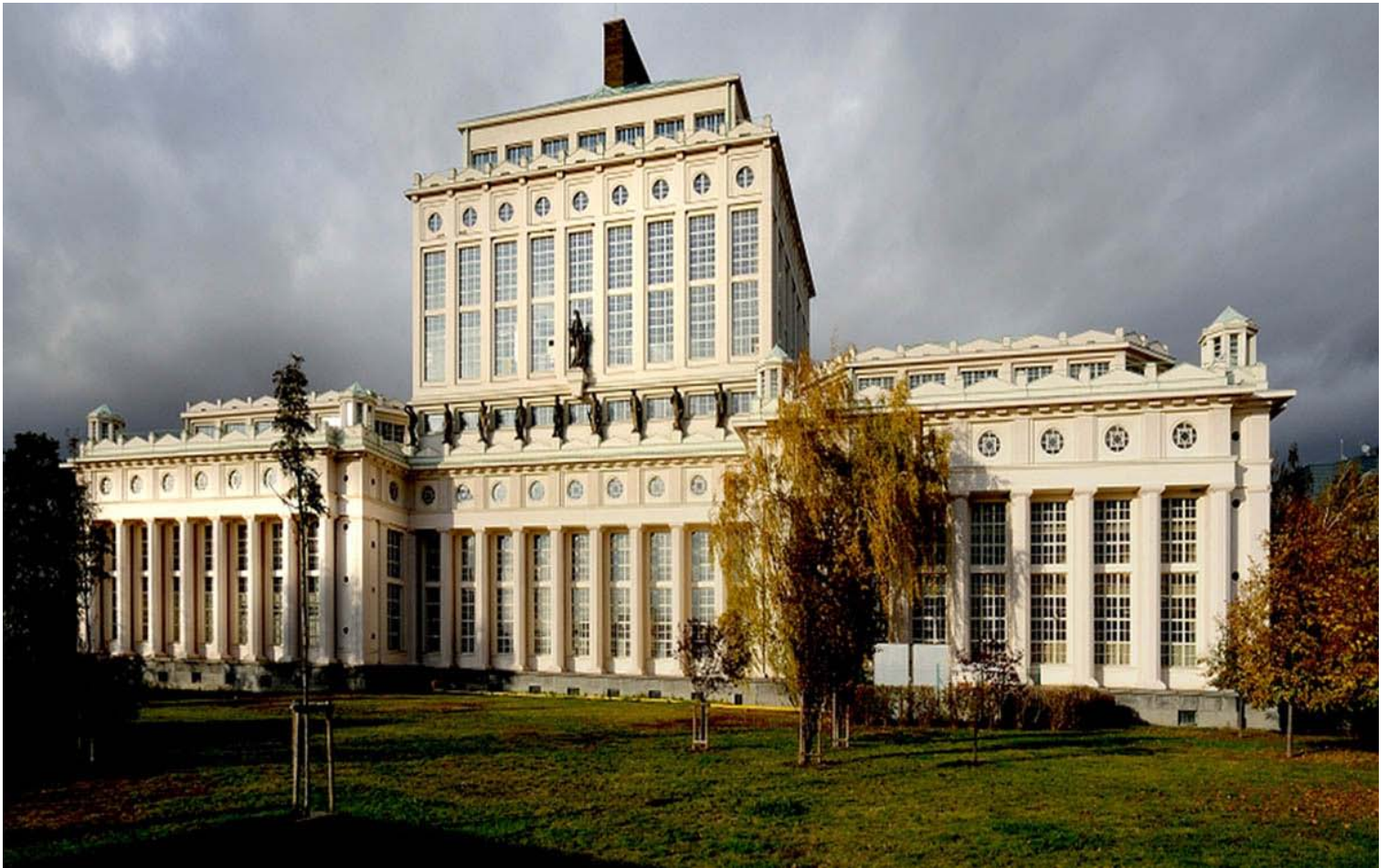
The Podolí treatment plant in Prague reflects the importance of water infrastructure for early 20th century urbanites. © PVK
