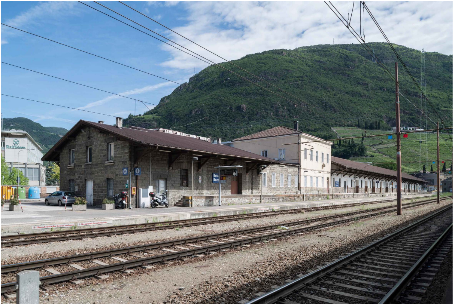
The track-side view of the Bozen railway freight shed, long enough to unload a whole train. © Jaist
